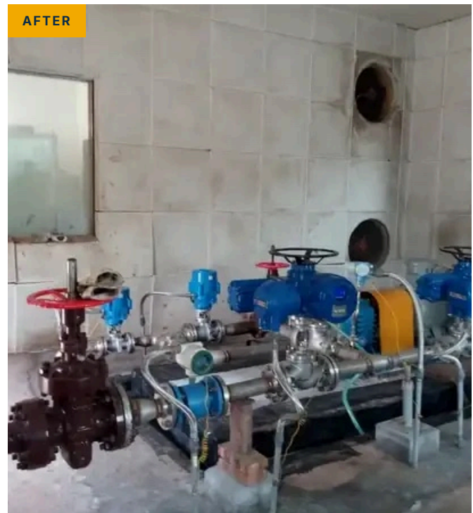
EHIK pitot tube pump · 45 kW (60 hp) motor
