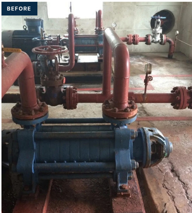
Before · Multistage pump, 90 kW (121 hp) motor
