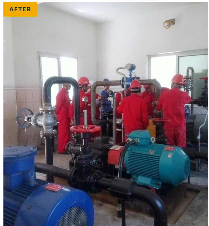
After · EHIK pump installation
