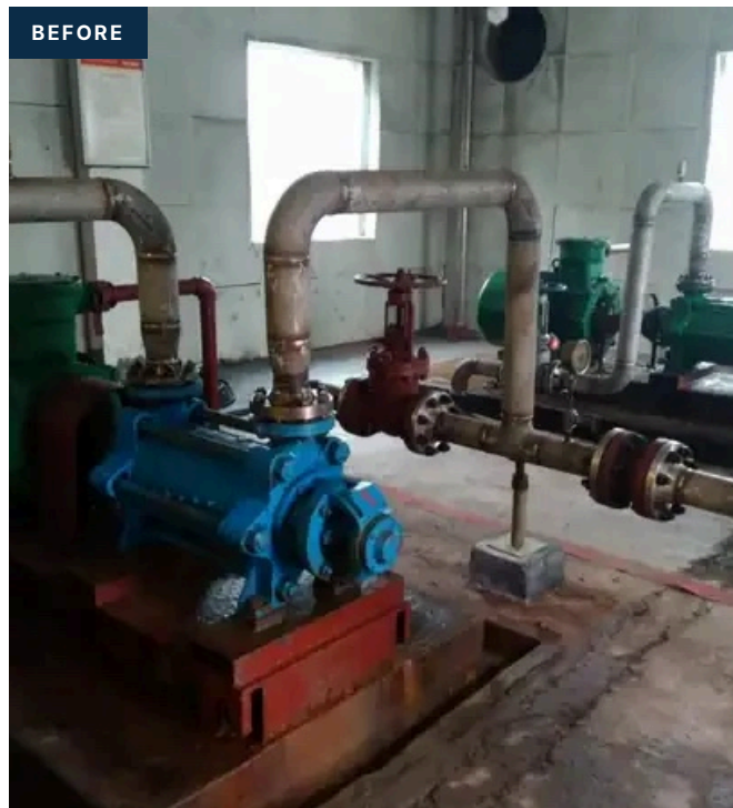
Multistage centrifugal pump · 90 kW (121 hp) motor
