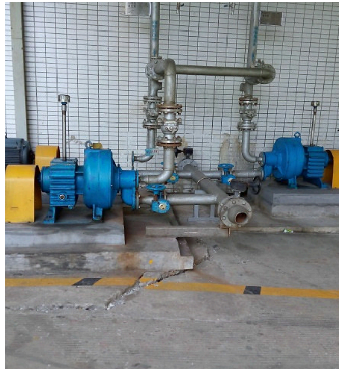
Vinda, China — shower-pump installation with the surrounding pipework and valves.
