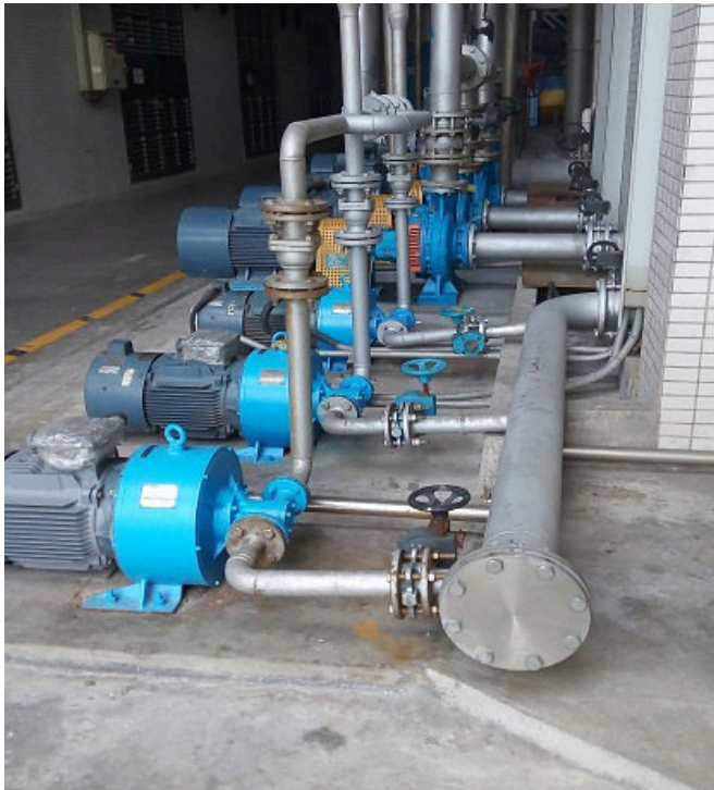
Felt and wire-screen shower pumps at a Vinda paper mill in China.
