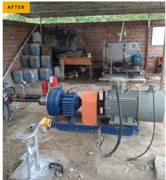
After · EHIK pump, 45 kW (60 hp) motor
