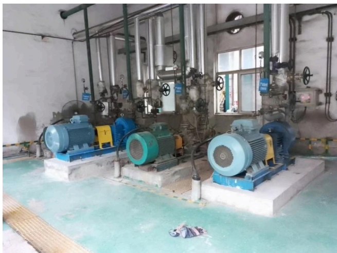
Pump installation at Jingbao Xinao Chemical.
