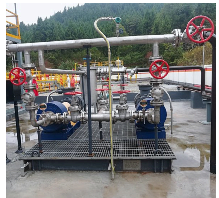
Installed on site
