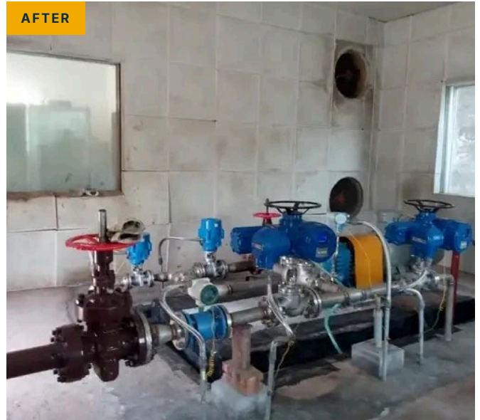
EHIK pitot tube pump · 45 kW (60 hp) motor
