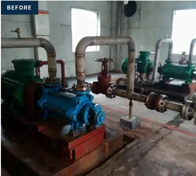
Multistage centrifugal pump · 90 kW (121 hp) motor
