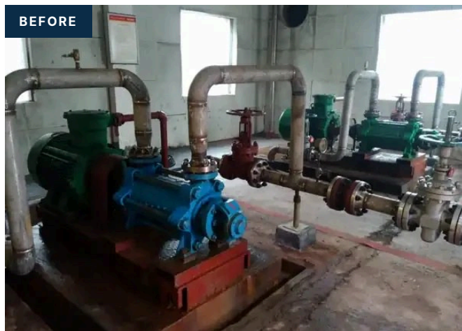
Multistage centrifugal pump · 90 kW (121 hp) motor
