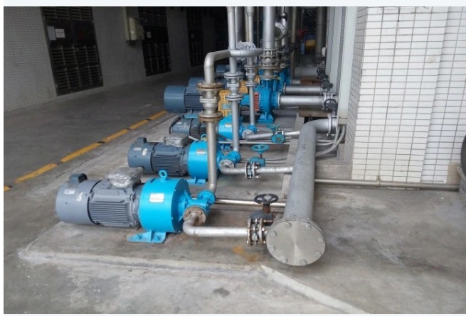
Felt and wire-screen shower pumps at a Vinda paper mill.
