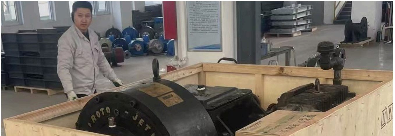
Roto-Jet pump at EHIK for a complete-pump overhaul.
