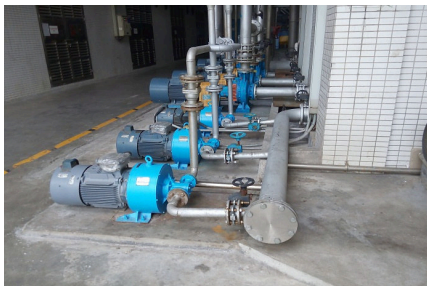
Felt and wire-screen shower pumps at a Vinda paper mill in China.
